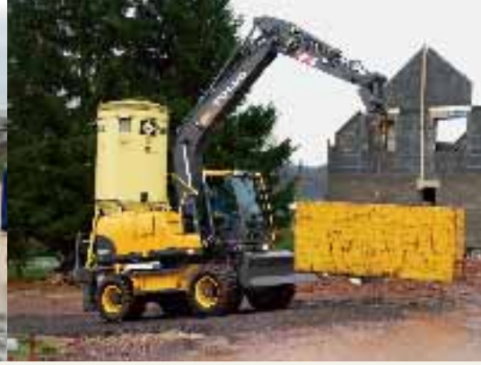
• Reach and power for lifting and placing.
