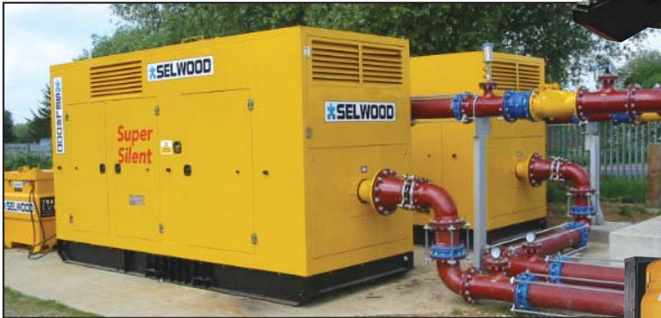
Flushing and priming of transfer main (UK)
